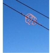
Bird Flight Diverters fitted to cables powering Rio Tinto's Oyu Tolgoi mine in Mongolia protect Houbara bustards and contribute to lender requirements and company targets.
